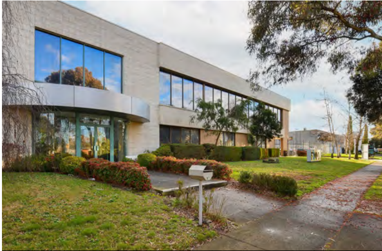
Major Capex Refurbishment 77-97 Ricketts Rd, Mt Waverly VIC
