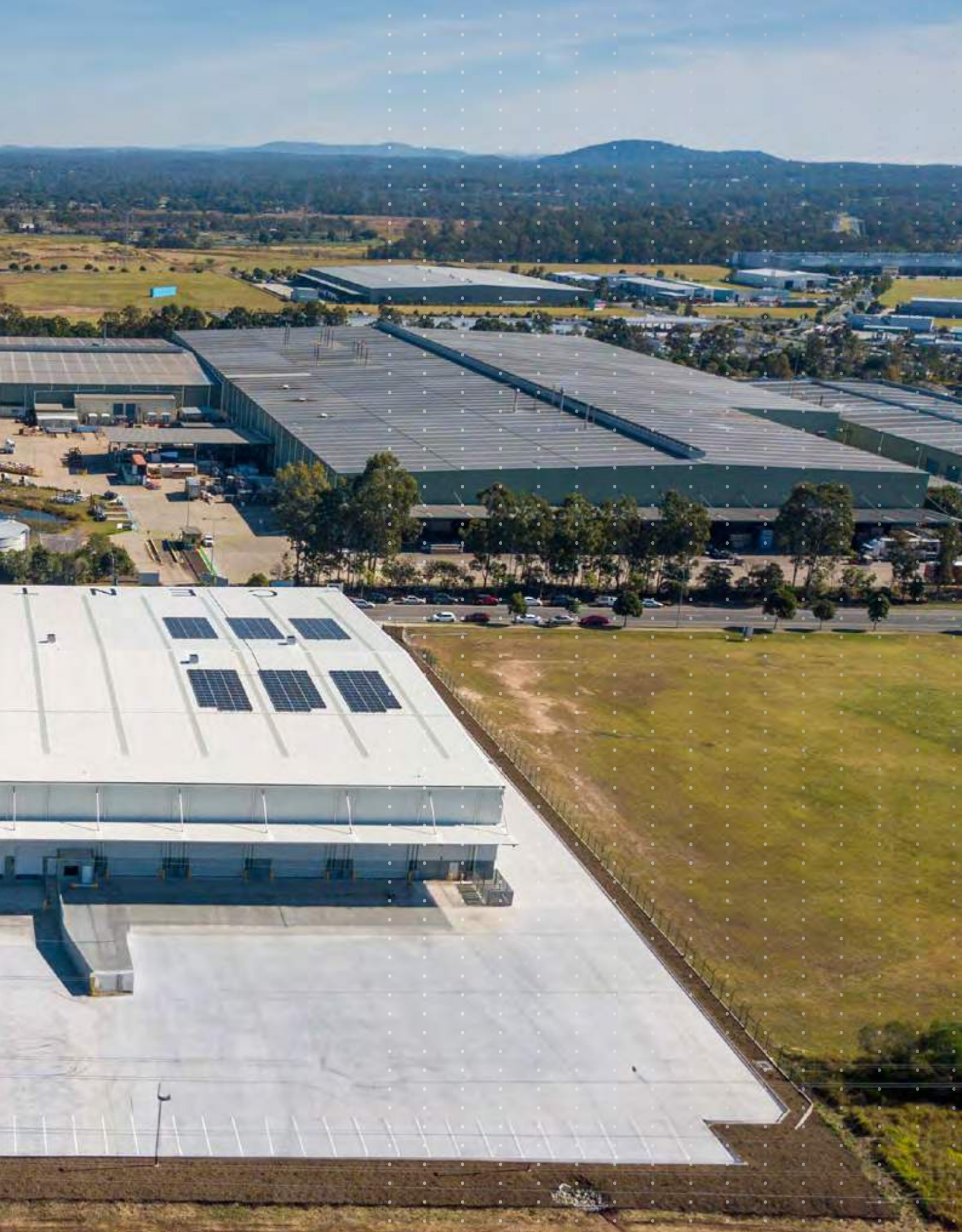
42 HOEPNER ROAD, BUNDAMBA QLD
